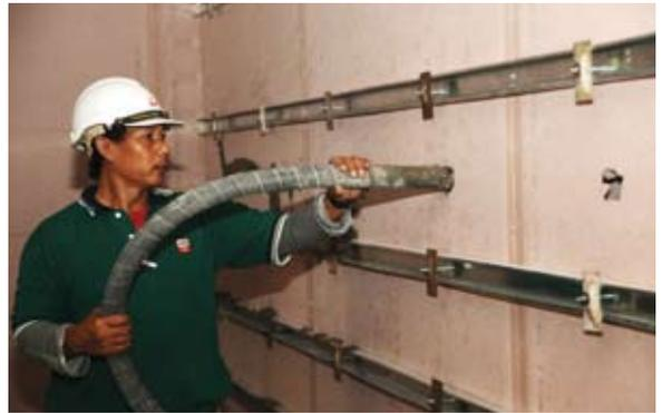
**STEP 6** The lightweight infill mix is pumped to each floor to fill the wall cavity.
