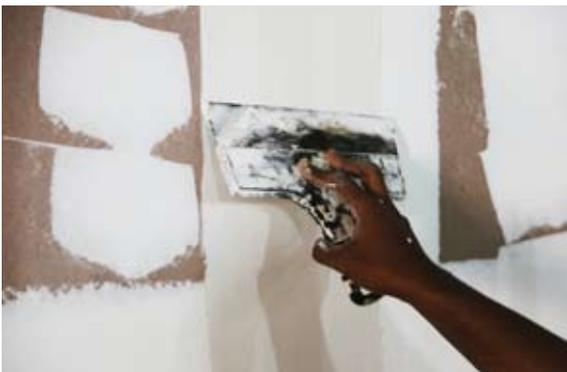
**STEP 7** Joint setting is done using the UCO Jointing Compound.
