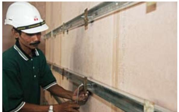
**STEP 4** Wall paneling is completed by fixing **UCO VISTABORD / UCO FLEXABORD** to the other side of the metal frame.
