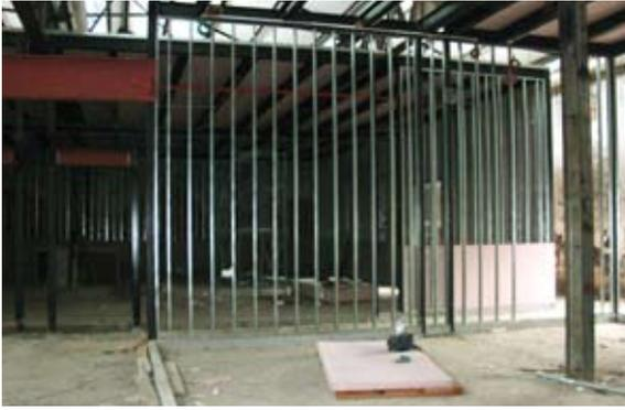
**STEP 1** Fix top metal track to structural support and bottom metal track onto the floor, thereafter light gauge metal stud frame is installed.
